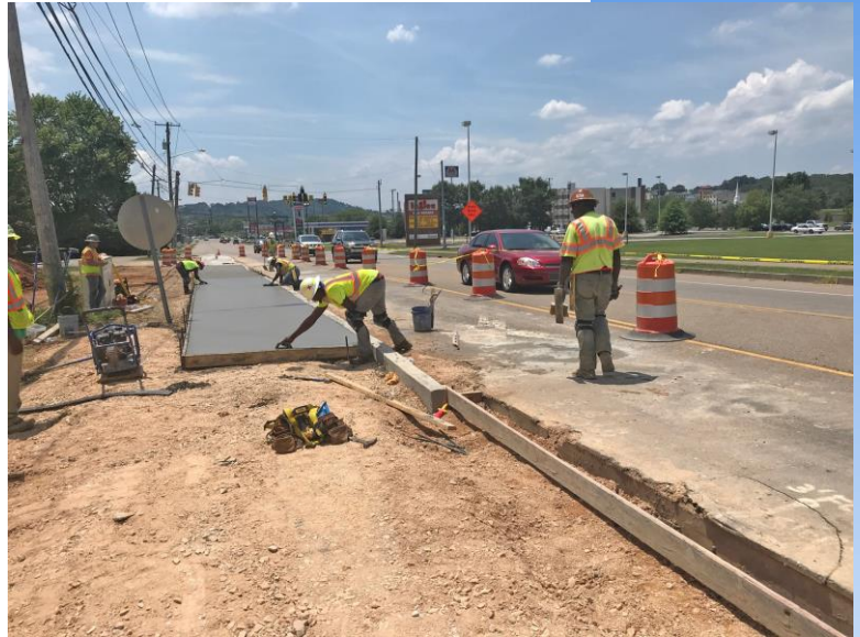
Cedar Lane Construction Looking West - July 2018
