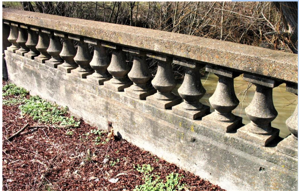
Existing Mineral Springs Avenue Bridge - Built in 1910
