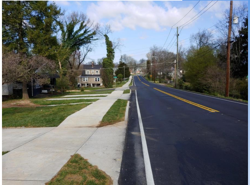
213 S Castle Street Looking North – Construction Complete
