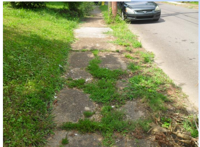
Portion of sidewalk within 2200 block of Edgewood Avenue to be replaced
