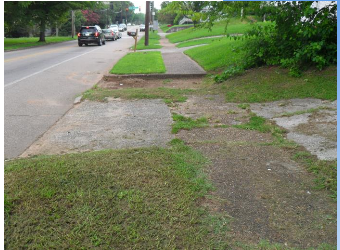
Portion of sidewalk within 2400 block of Cecil Avenue to be replaced
