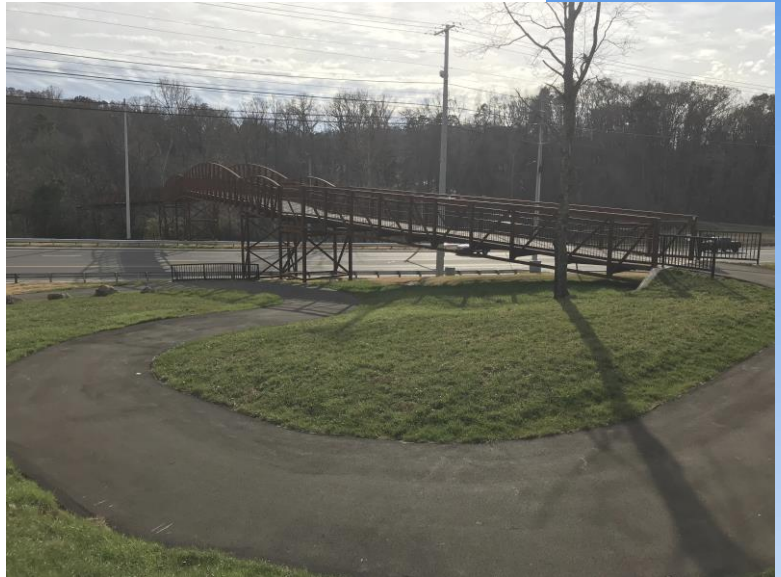
December 2018 - Construction Complete
