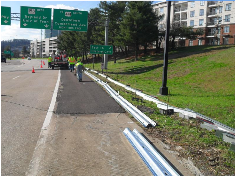
During Construction – March 2017
