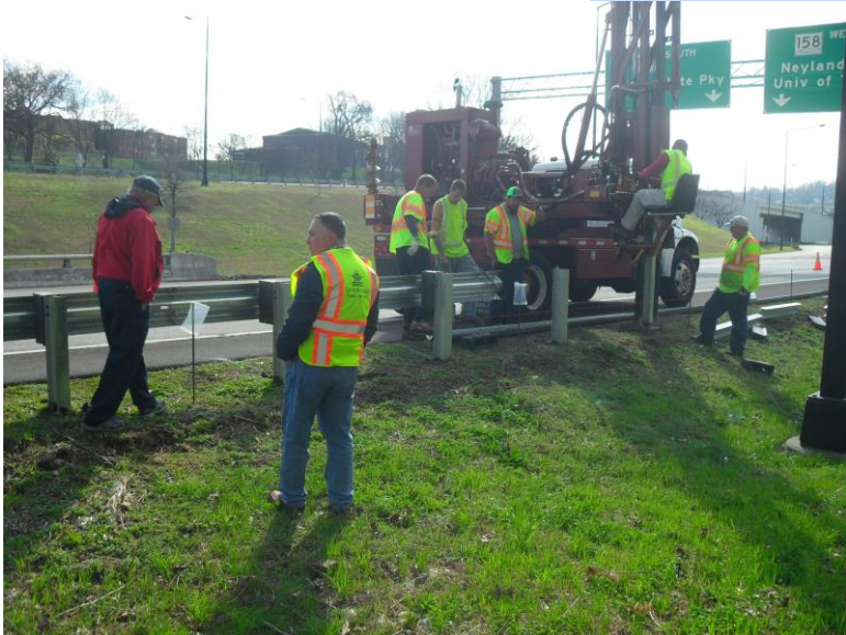
During Construction – March 2017
