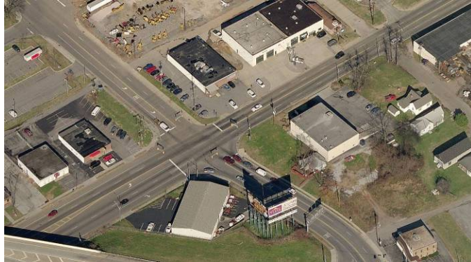
Middlebrook Pike from Twenty-First Street to Citico Street (Before Construction)
