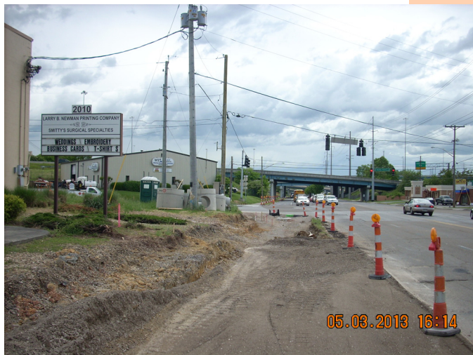
Middlebrook Pike at Twenty-First Street Looking West – During Construction
