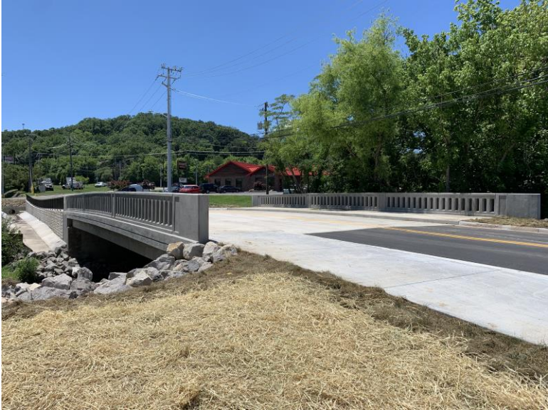
Construction Complete – June 2021
