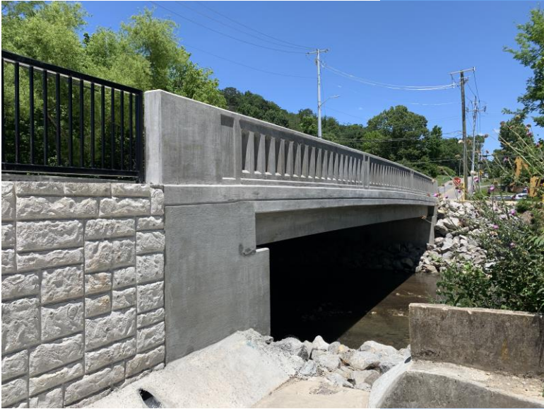
Construction Complete – June 2021
