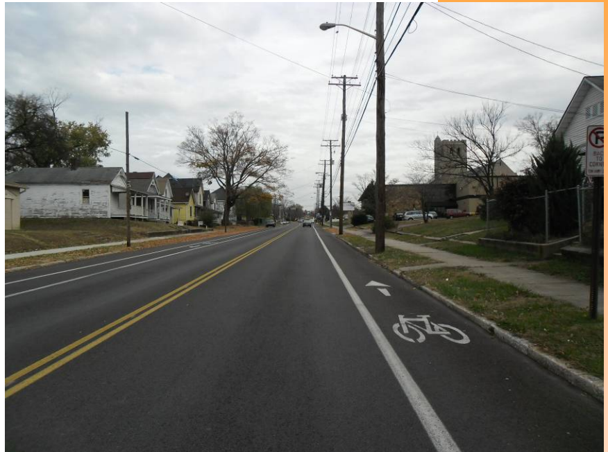
New Pavement Along Baxter Avenue
