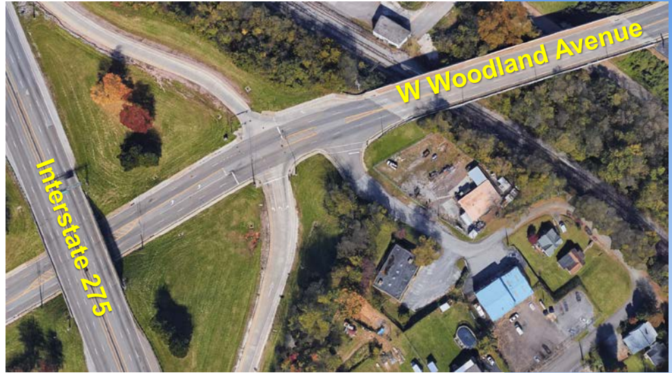
Woodland Avenue Bridge
