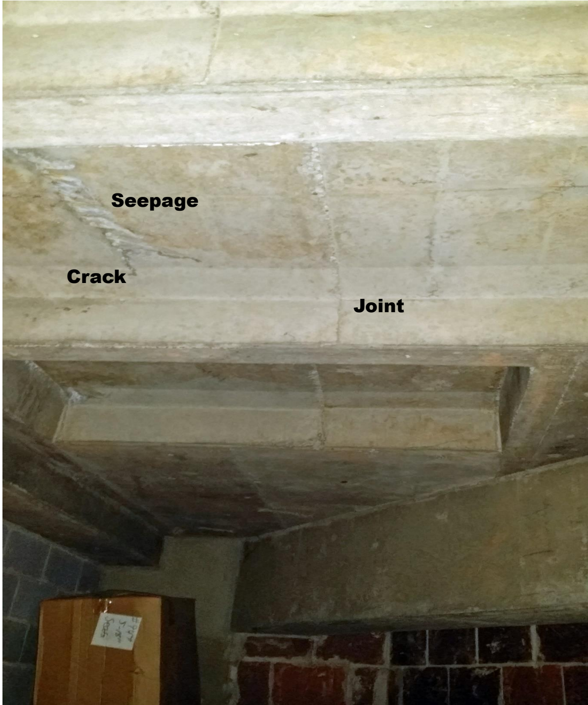
West Storage Area Ceiling
