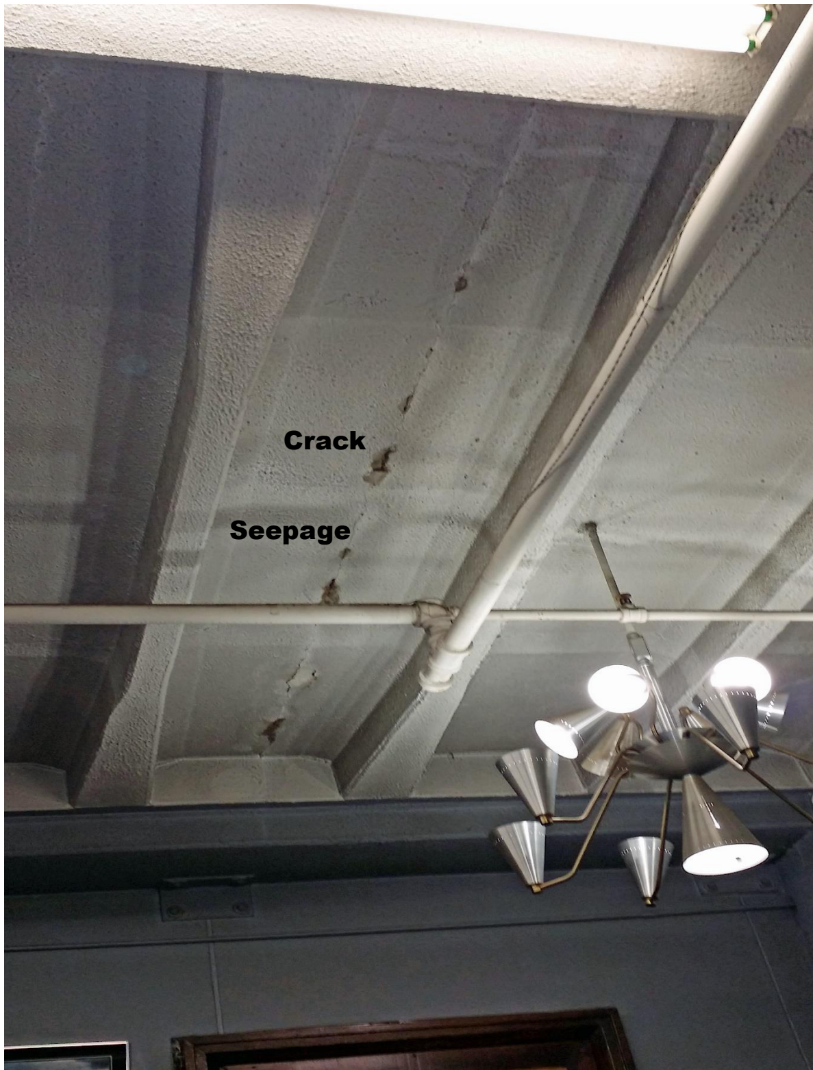
Stage Waiting Area Ceiling
