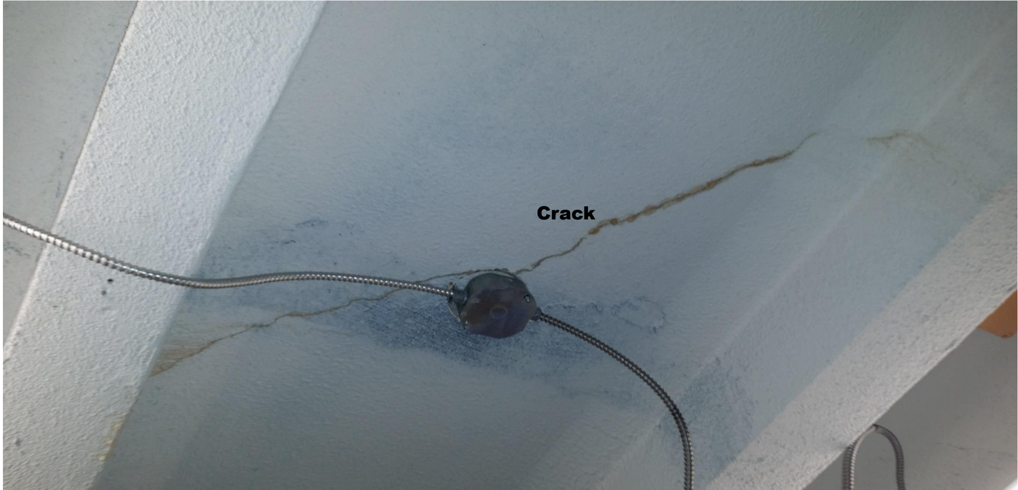
Ladies' Makeup Room Ceiling
