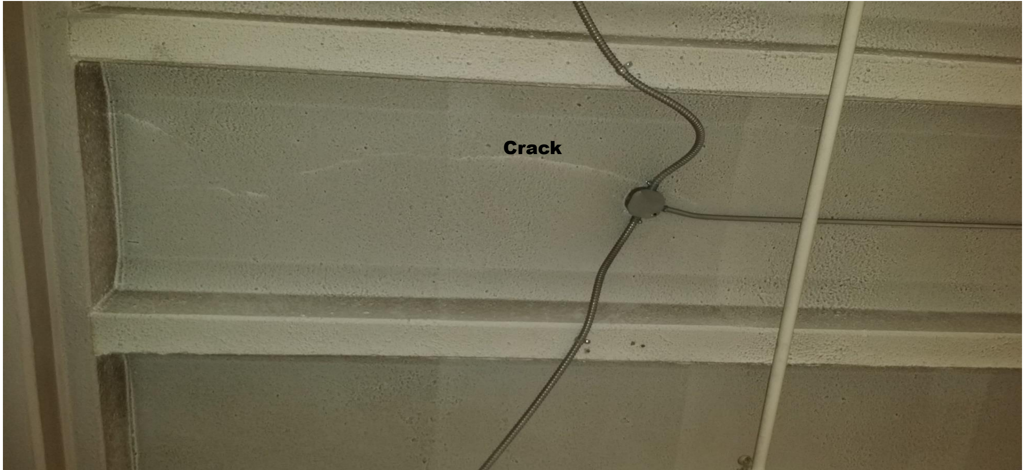
Stage Waiting Area Ceiling
