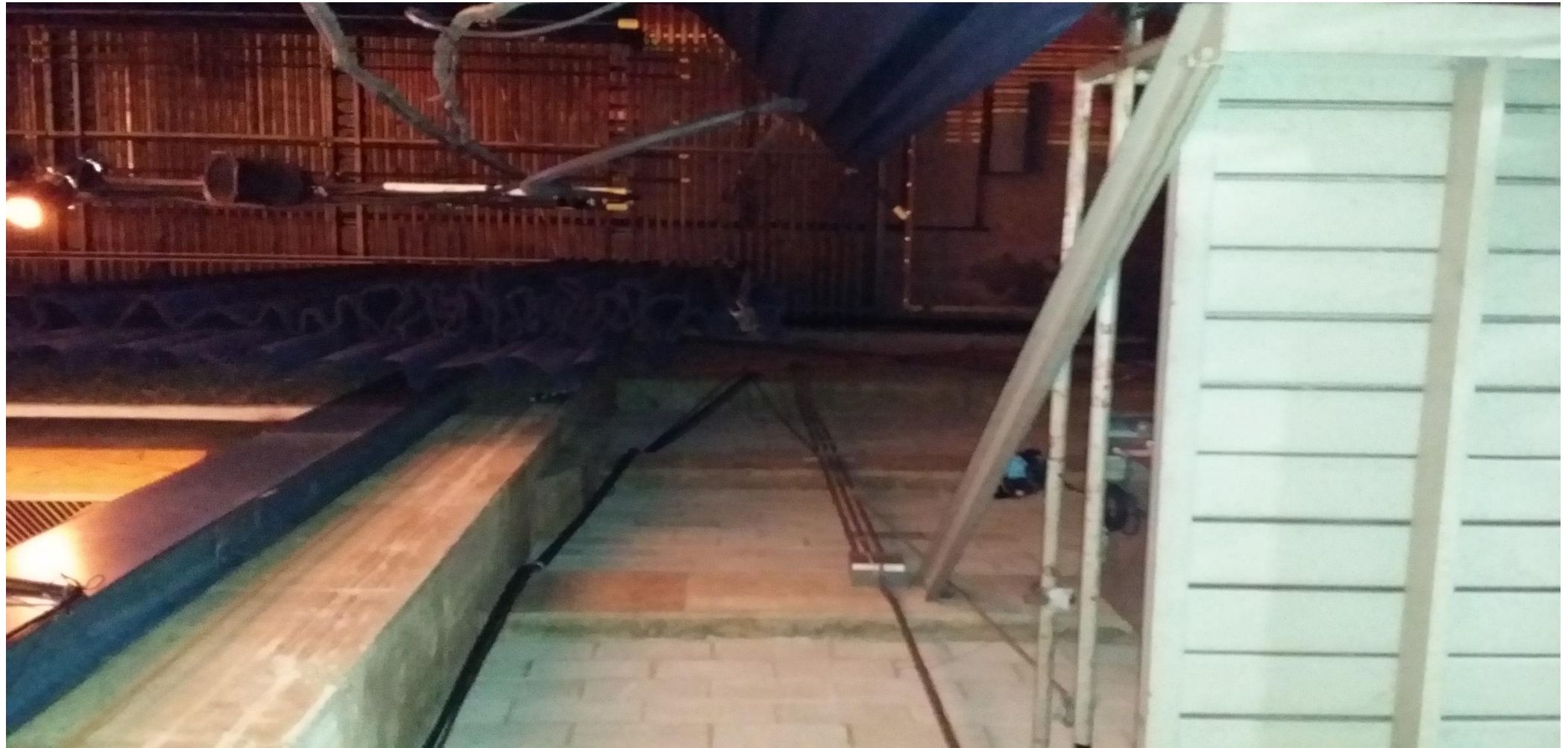
Stage South Wall
