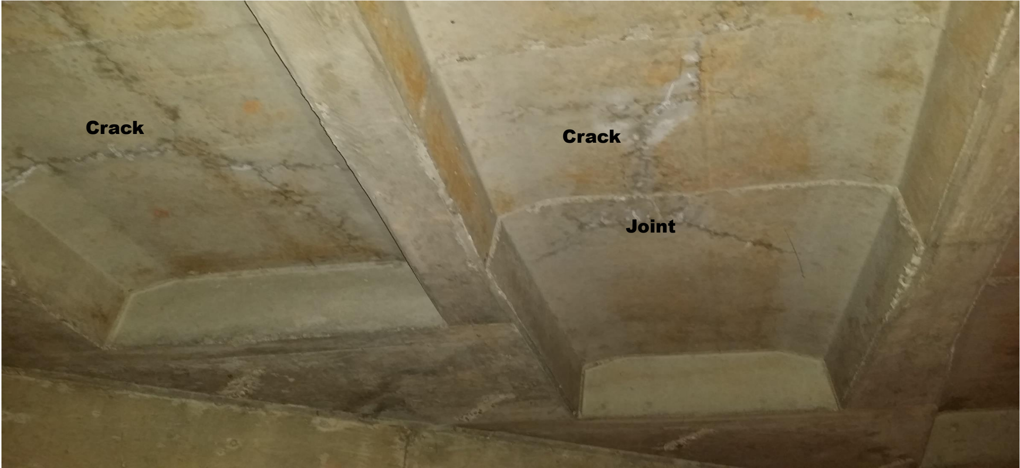
West Storage Area Ceiling
