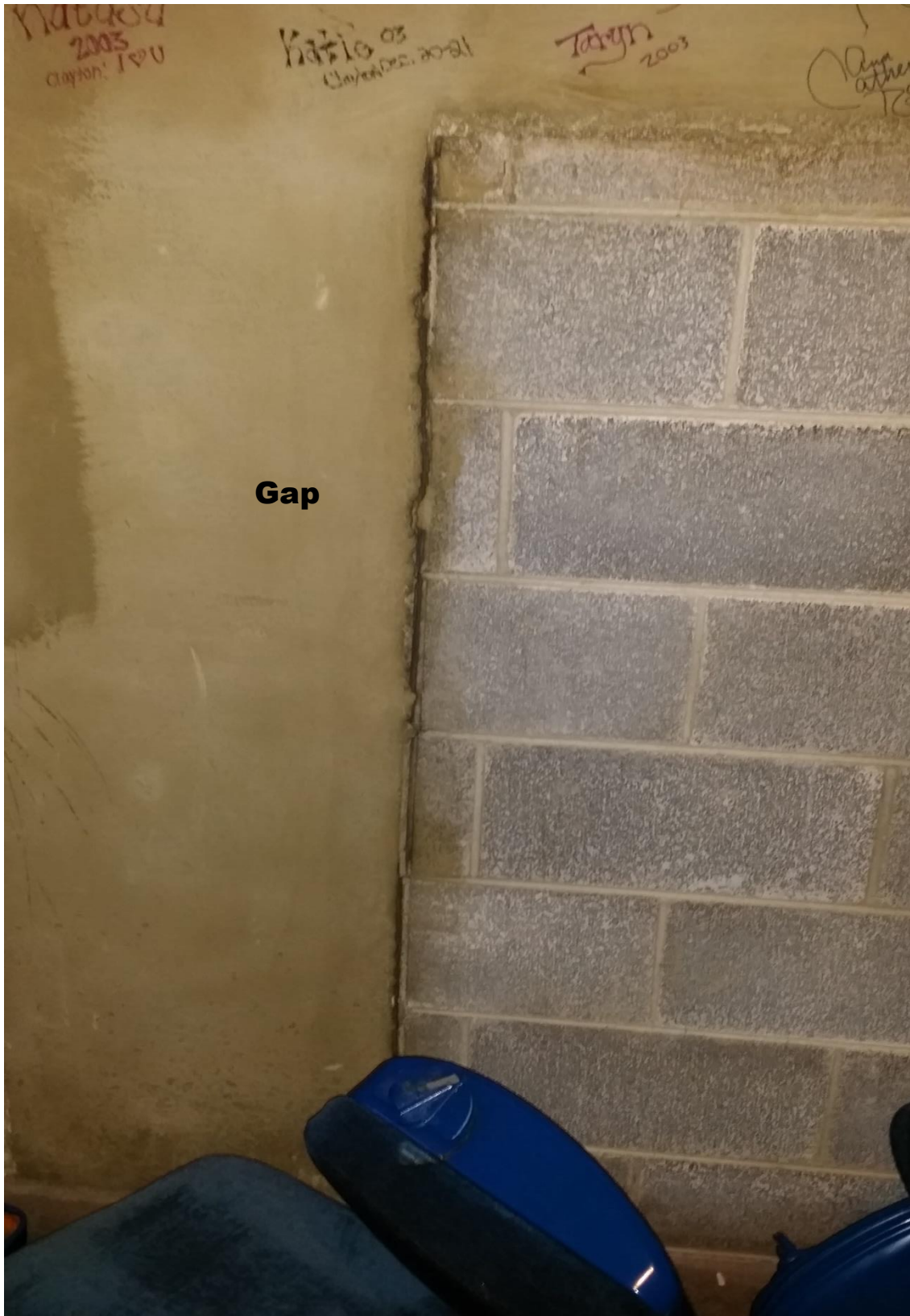
West Storage Area Wall
