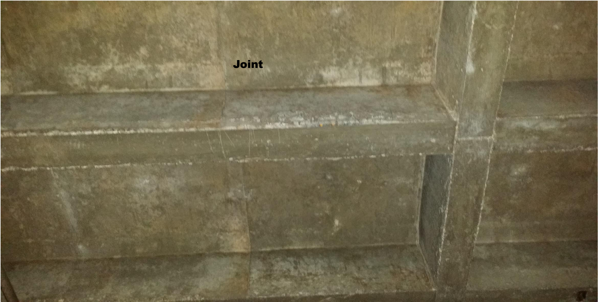
Stage Storage Room Ceiling
