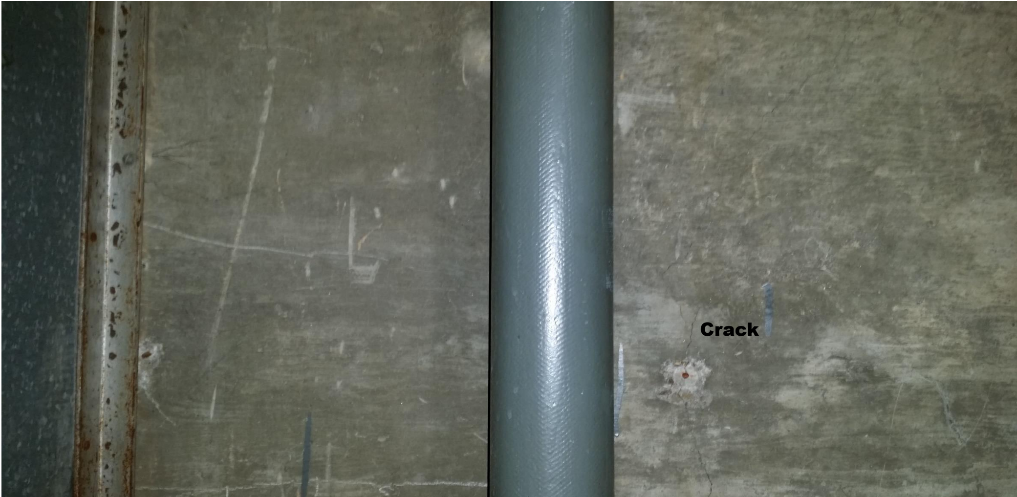
Mechanical Room Wall
