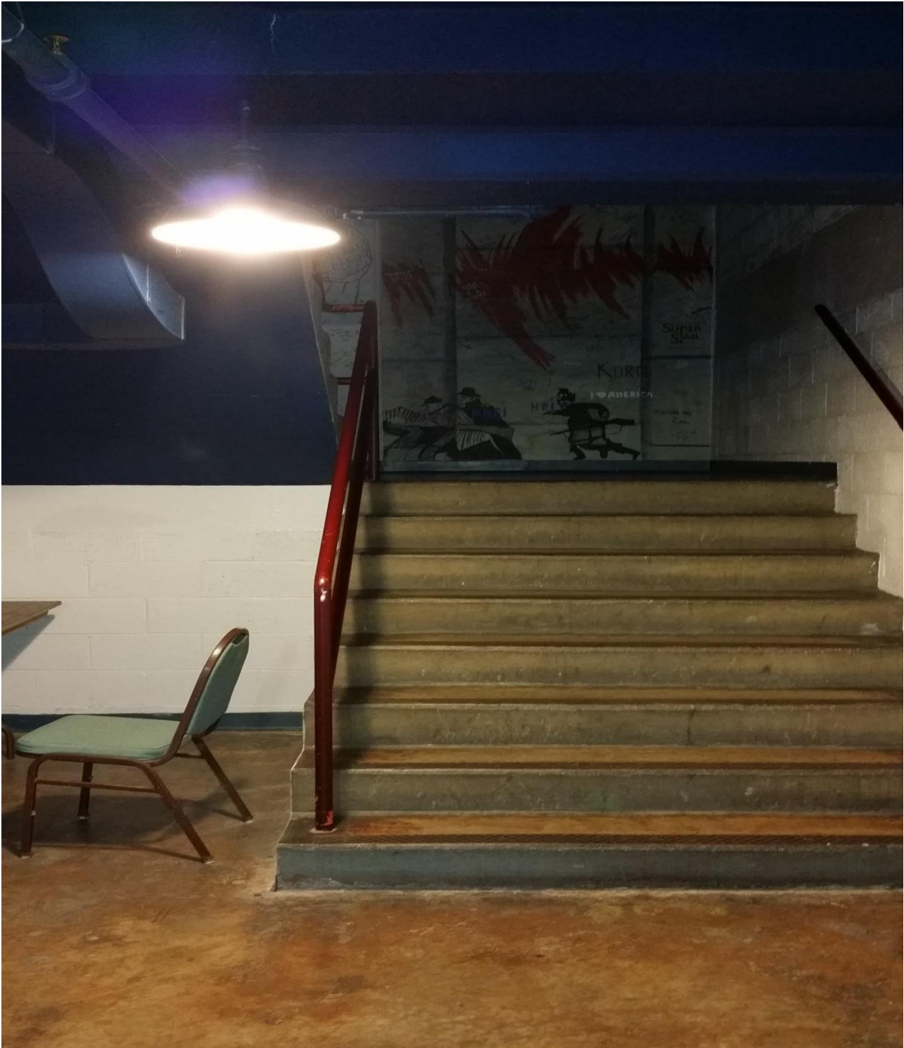
West Stair leading to Dressing Room
