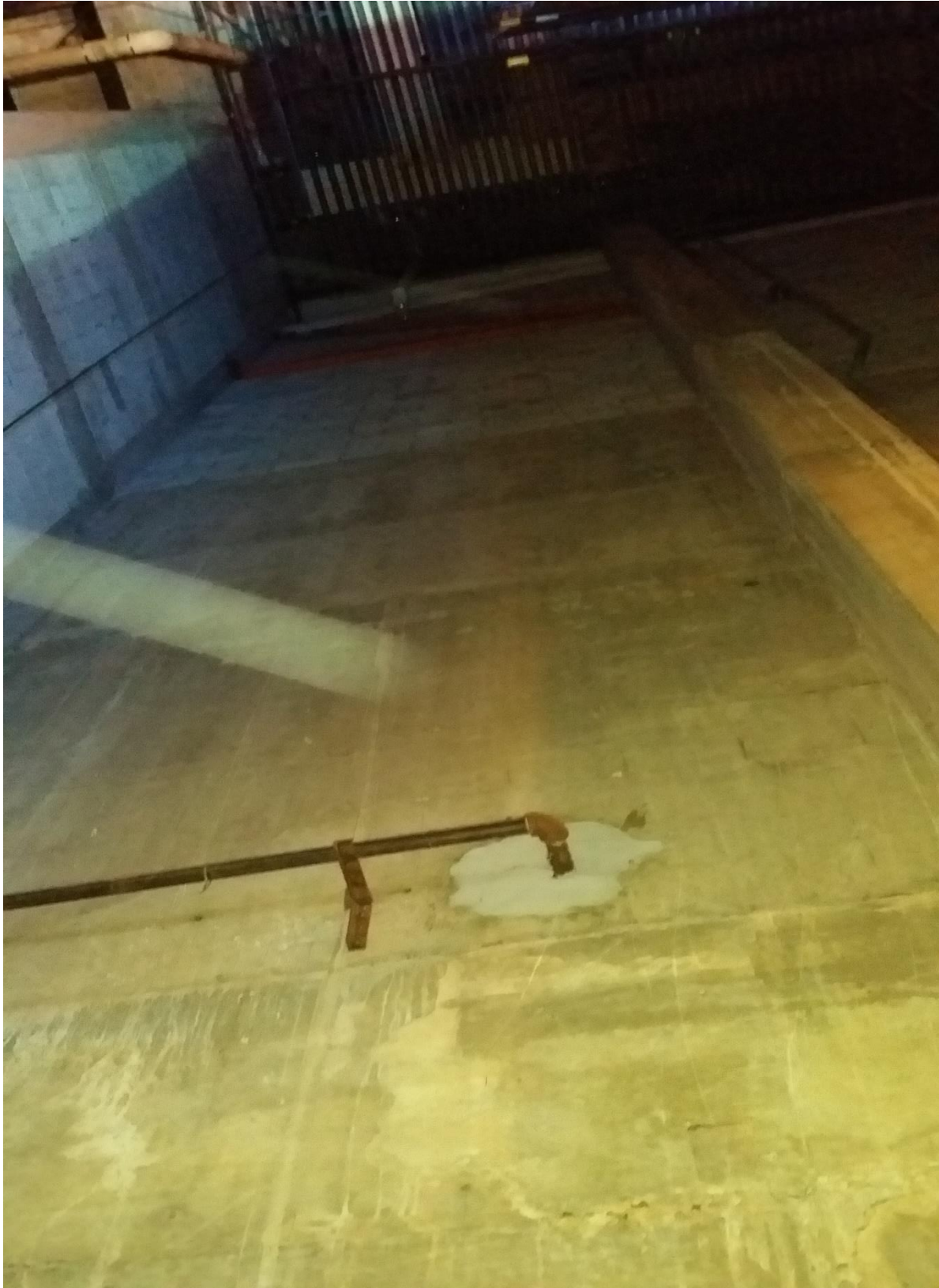
Stage South Wall
