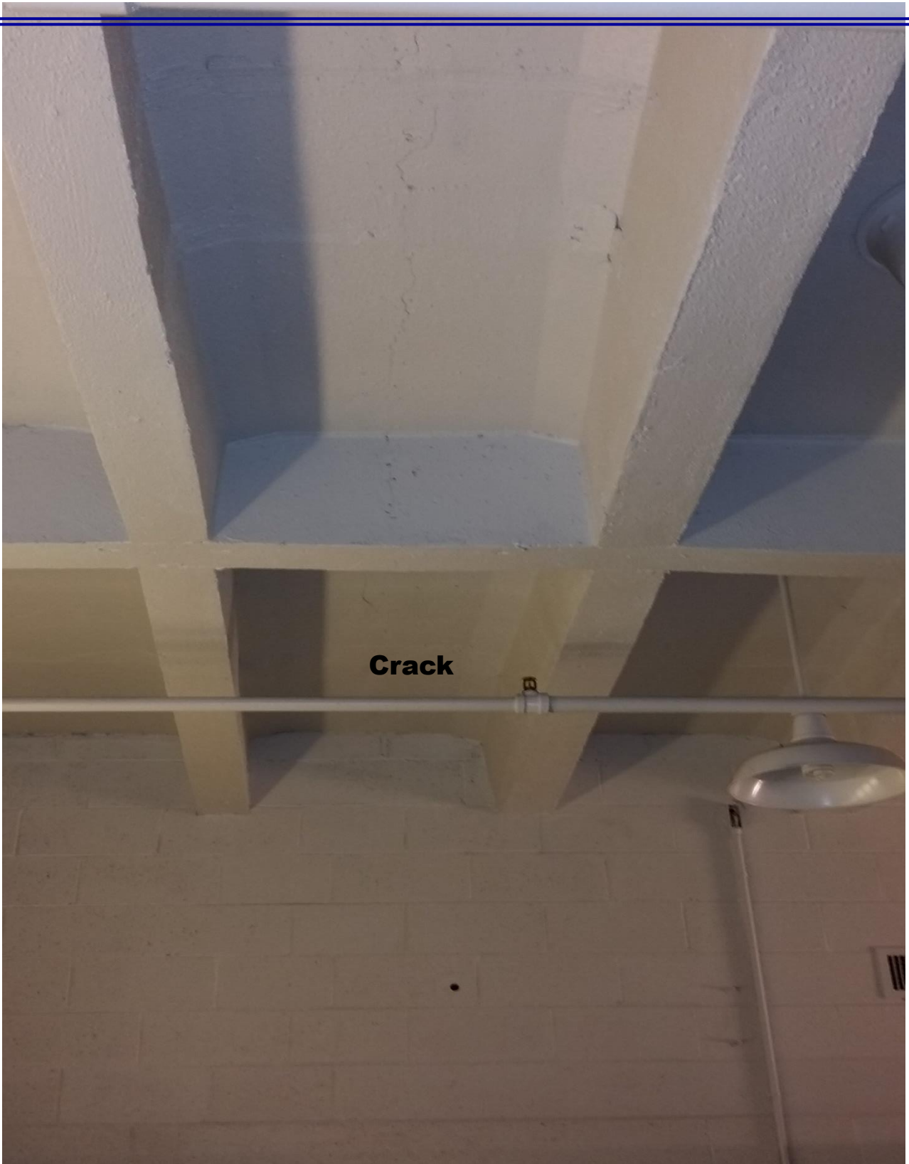
Men's Makeup Room Ceiling
