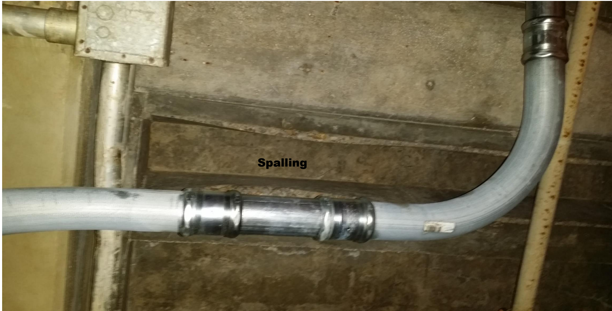
Stage Storage Room Ceiling
