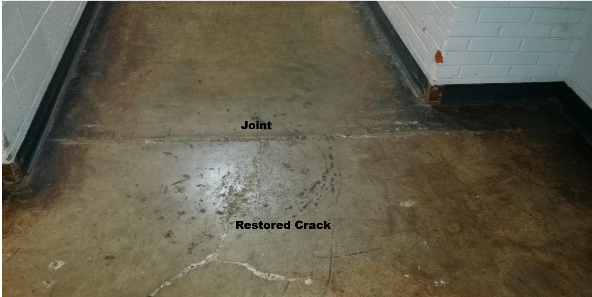
Landing Floor at East Stair
