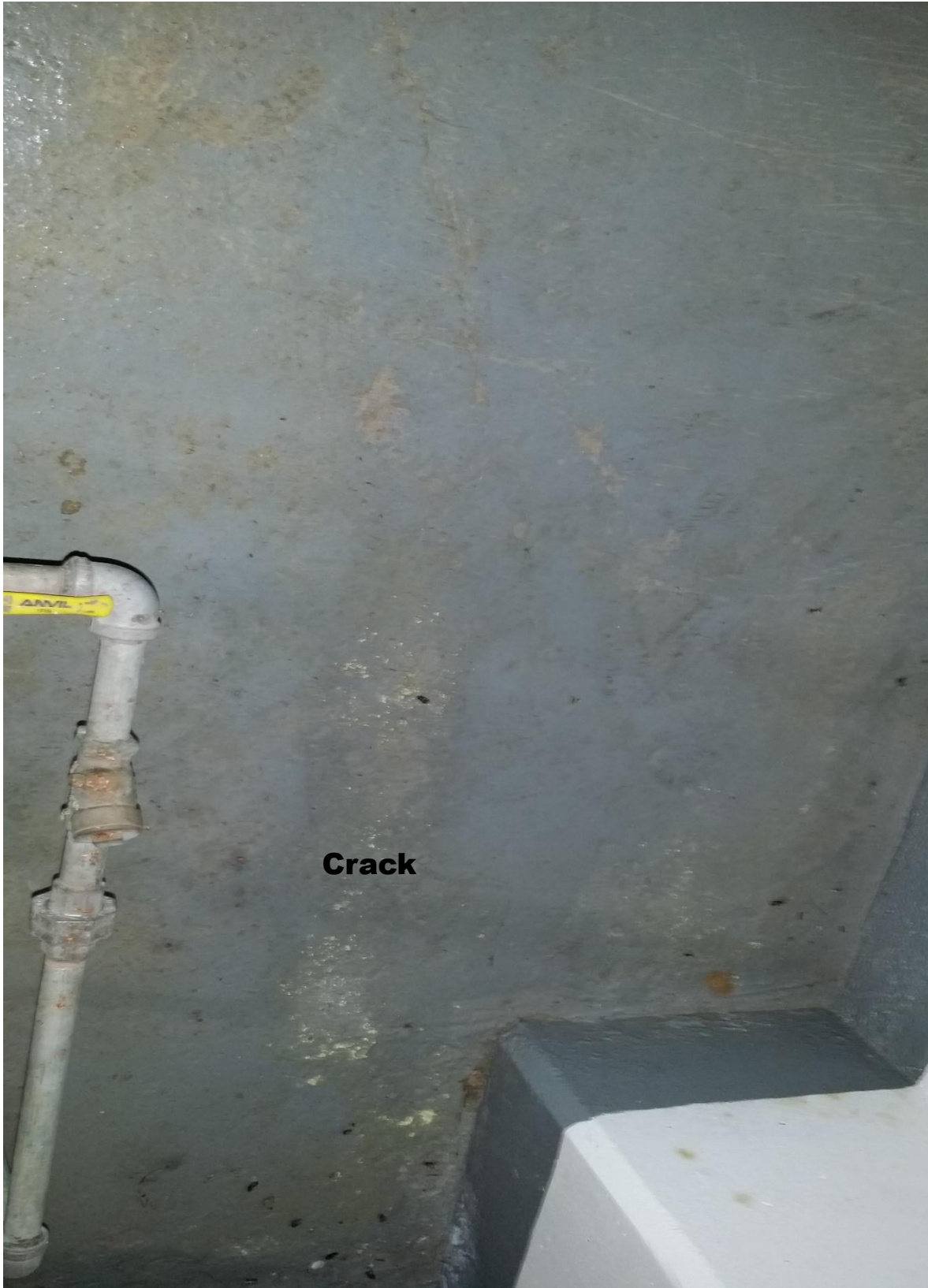
Boiler room Floor
