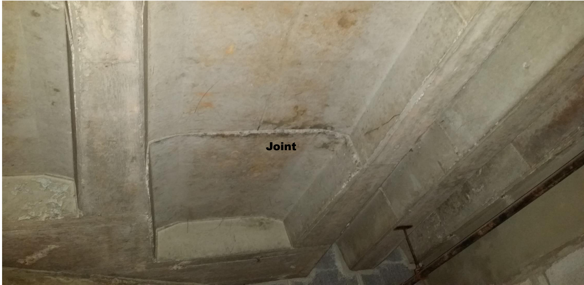
West Storage Area Ceiling
