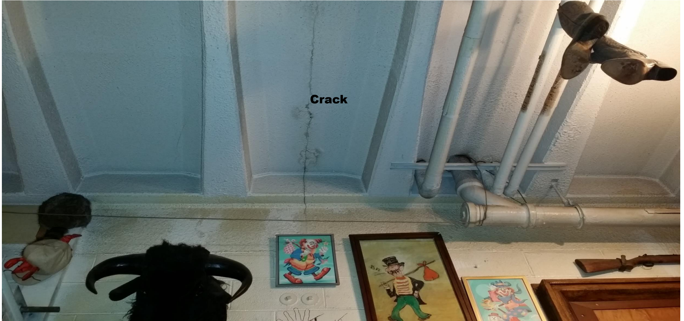
Stage Waiting Area Ceiling
