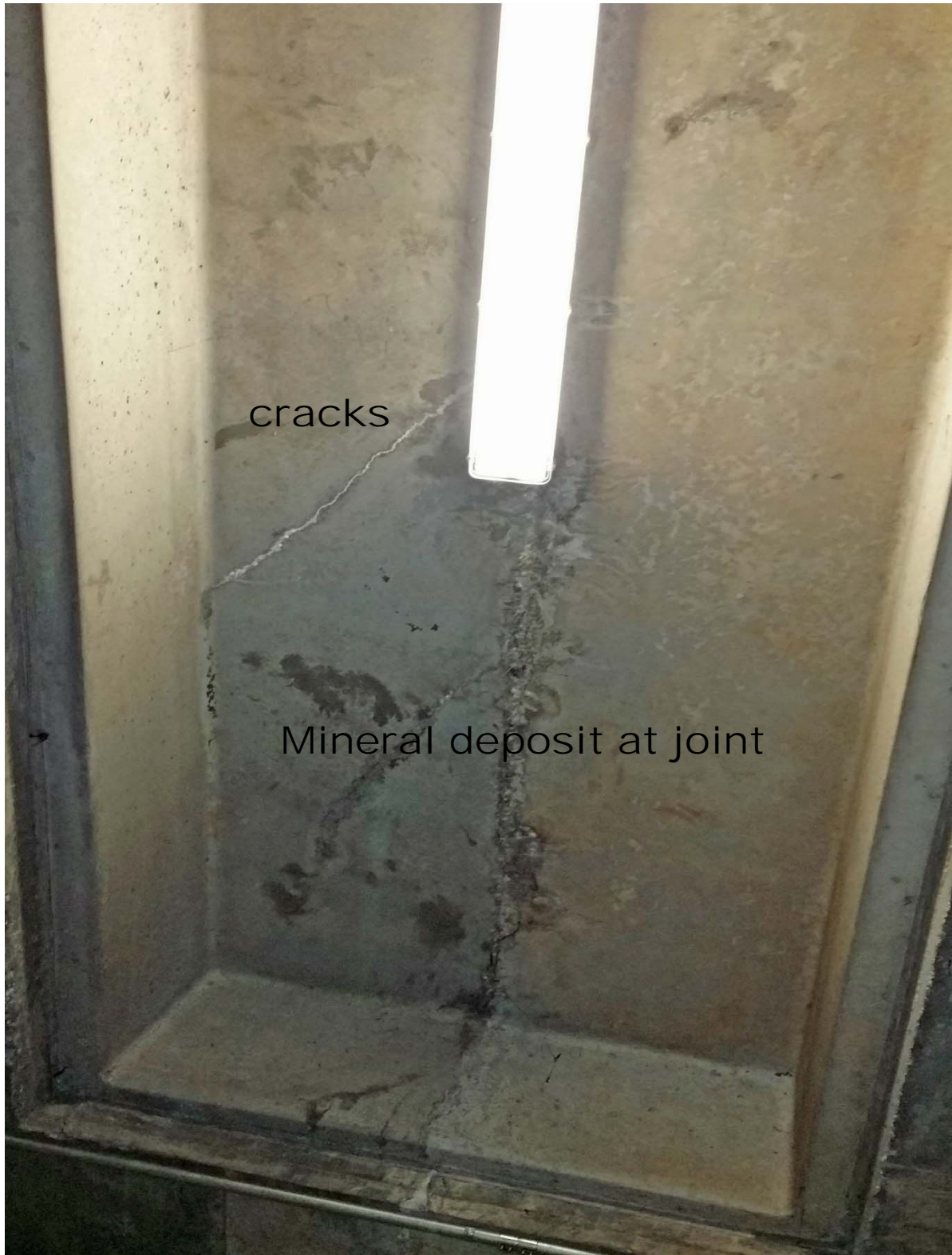
Service Garage Ceiling
