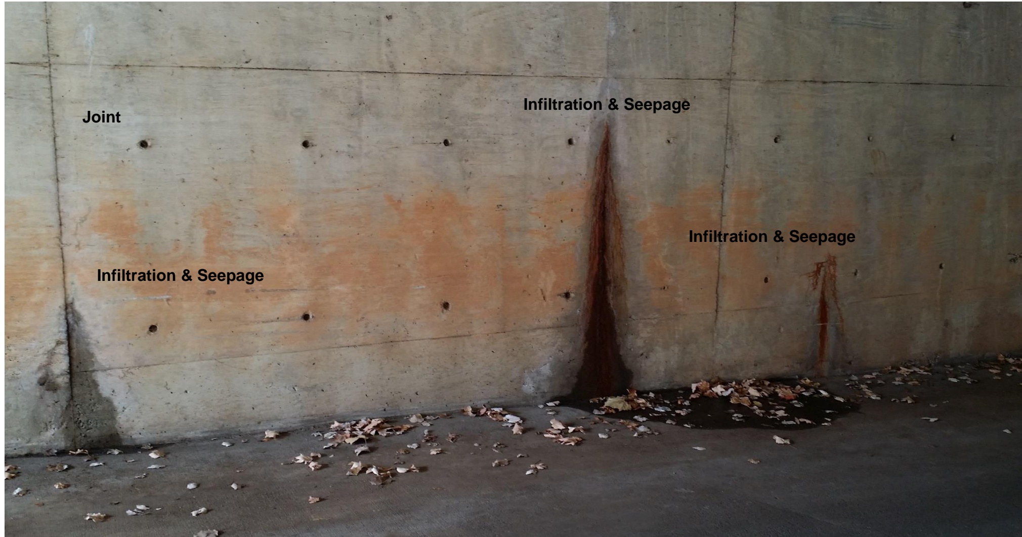
Ramp West Wall
