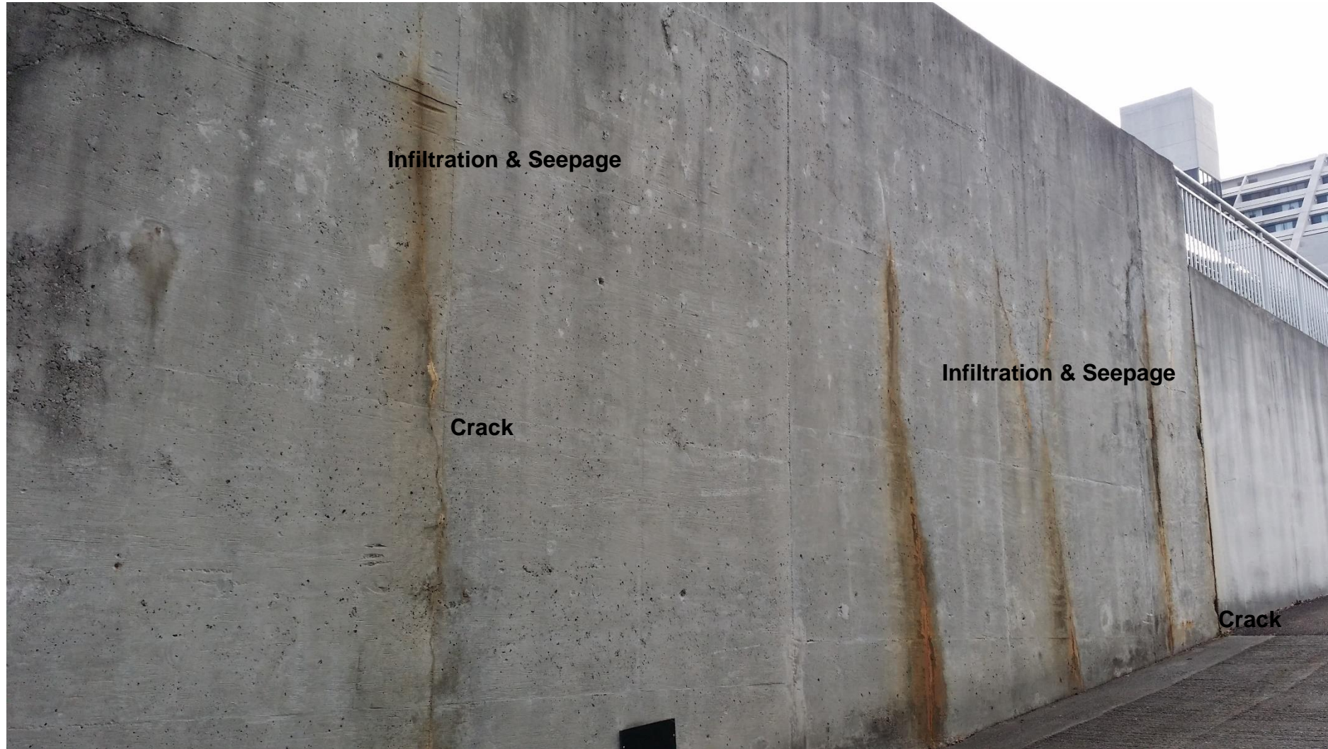
Ramp east wall
