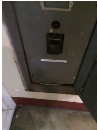
E.6 Electrical Panel cover not fitting properly and wires exposed.
