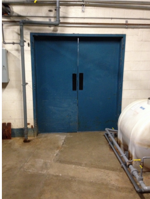
M.19 Ice Chiller Room doors
