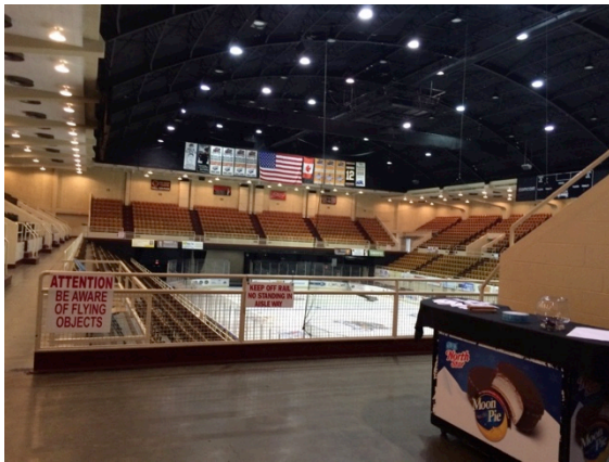
E.18 Sports Lighting for Coliseum
