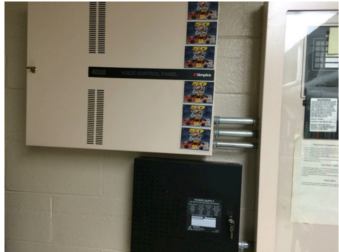
E.20 Fire Alarm Control Panel
