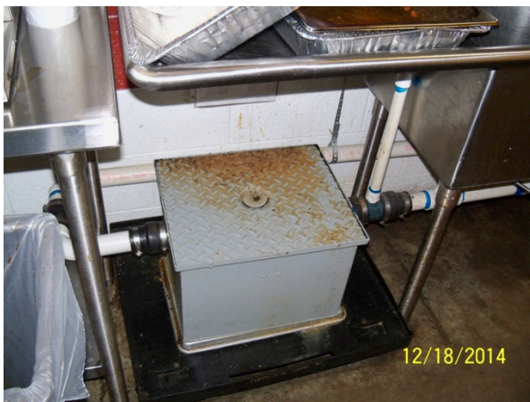
P.18 Grease trap in one of the many concession stands
