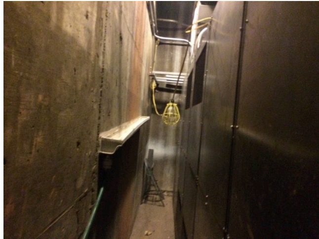
E.6 Electrical Panel cover not fitting properly and wires exposed.
