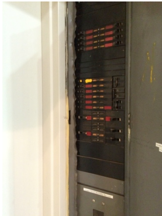
E.5 Electrical Panel Showing Considerable Wear.
