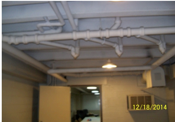
P.5 Screwed galvanized waste and vent piping material
