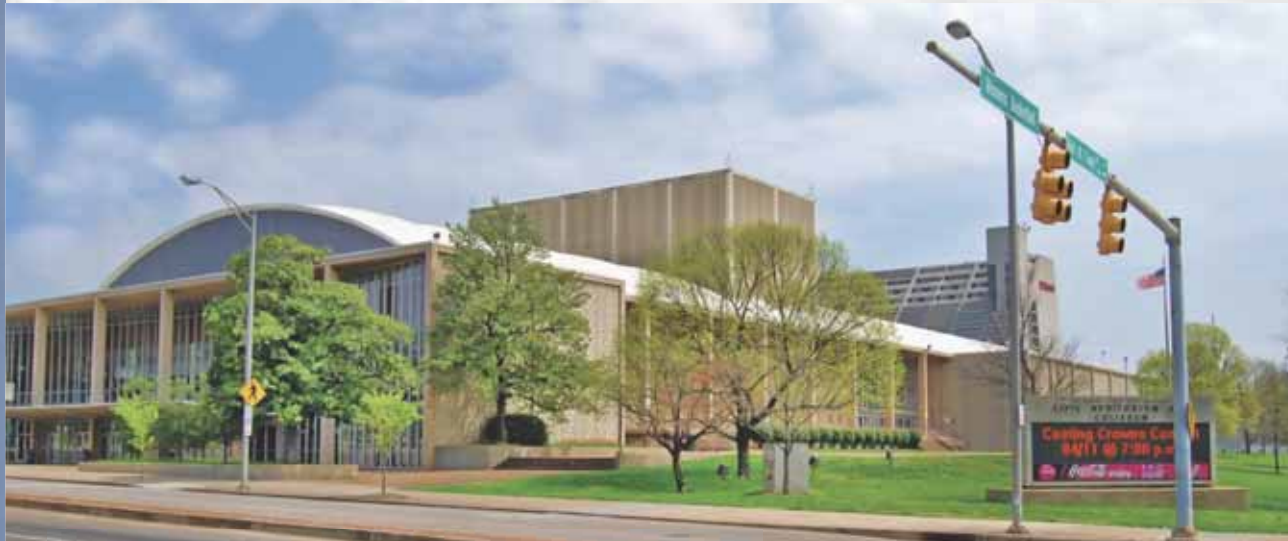
Knoxville Civic Auditorium and Coliseum
