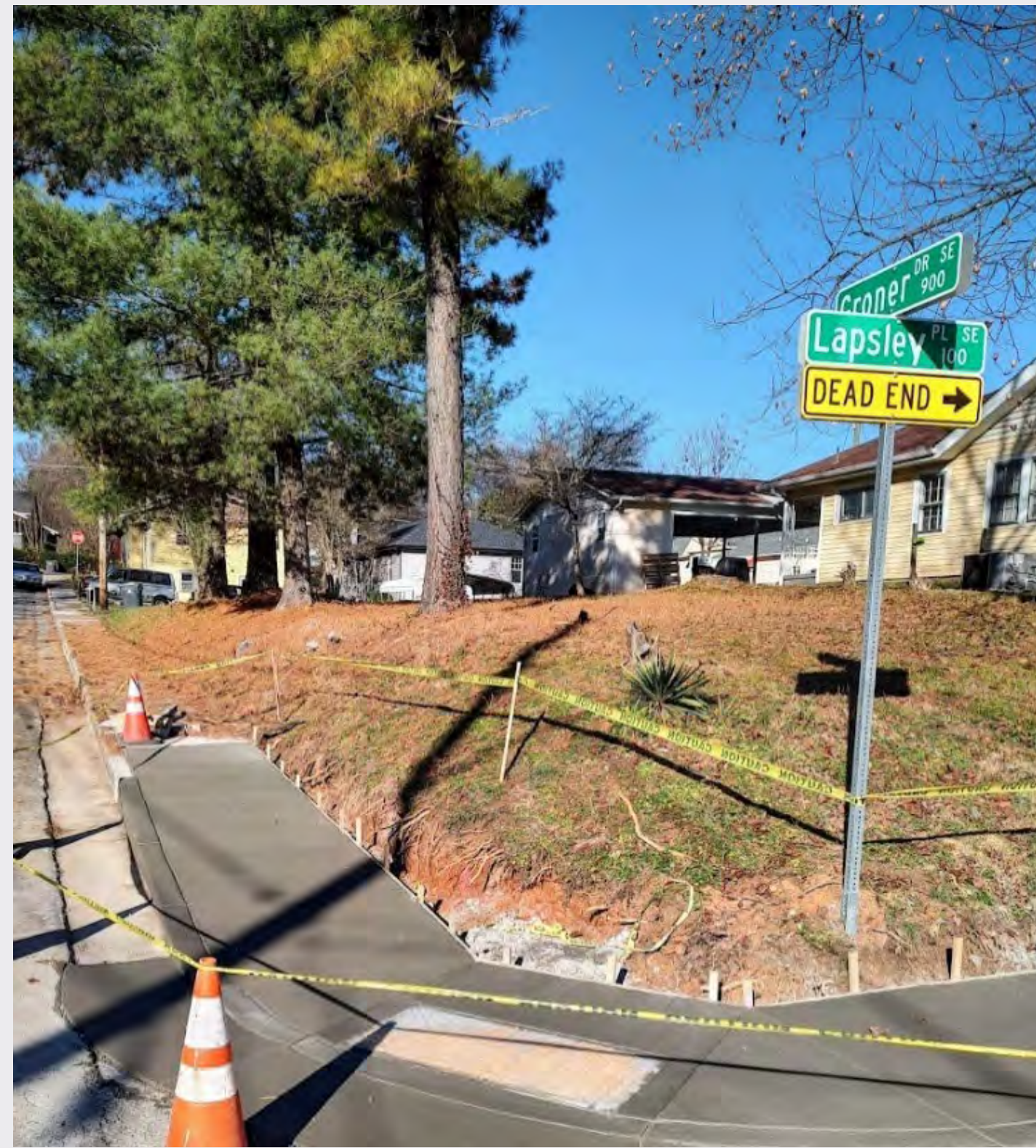
Sidewalk Replacement at Groner Drive and Lapsley Place
