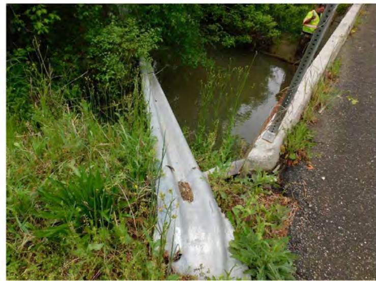
GUARDRAIL REMOVED (RT) - APPROACH 2
