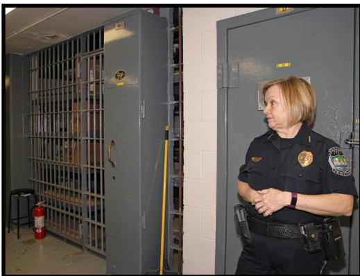
Original jail floor, now used for storage
