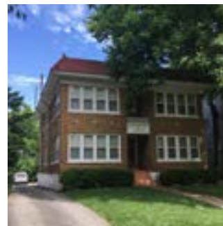
Figure 2.11 Example of engaged stoop MMH frontage. Multiple units in the building are accessed by a single, shared entry that leads to a hall or small lobby area.
