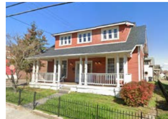
Duplex Side-by-Side (MMH) 2 units Knoxville, TN
