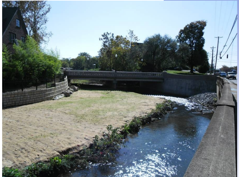
Fairmont Bridge Construction Complete
