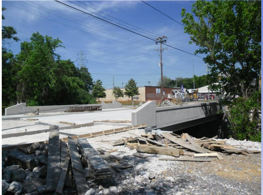
Glenwood Avenue Bridge - During Construction
