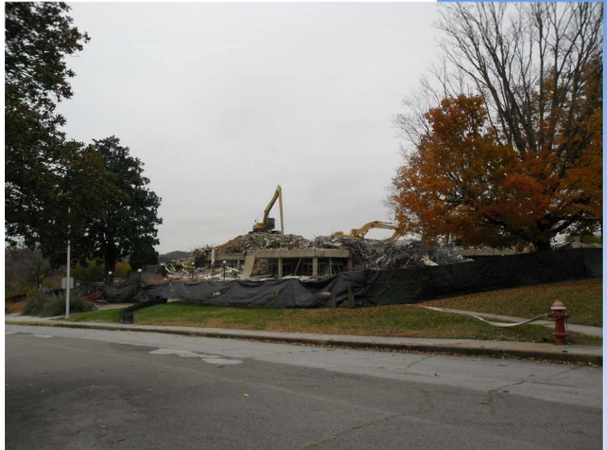
Demolition of Chota Building November 2014
