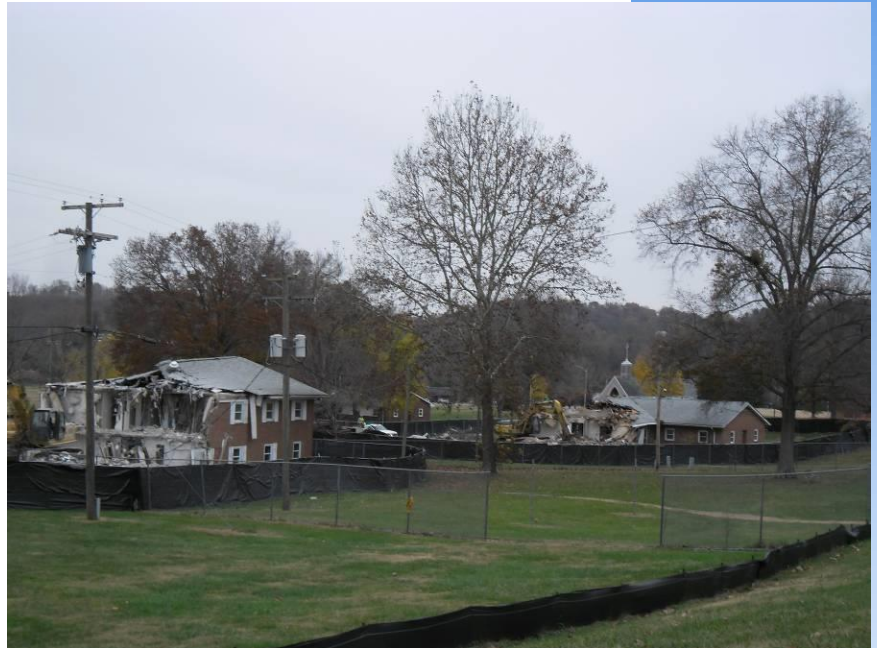
Demolition of Magnolia Cottage and Cherry Cottage November 2014
