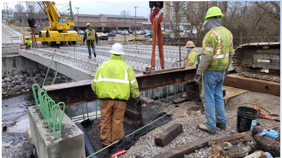
During Construction – February 2021
