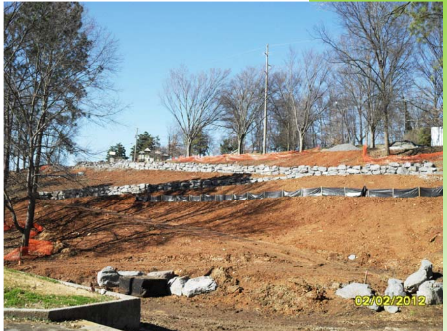
Morningside Park During Construction
