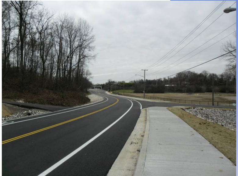
Construction Complete – Looking Northwest
