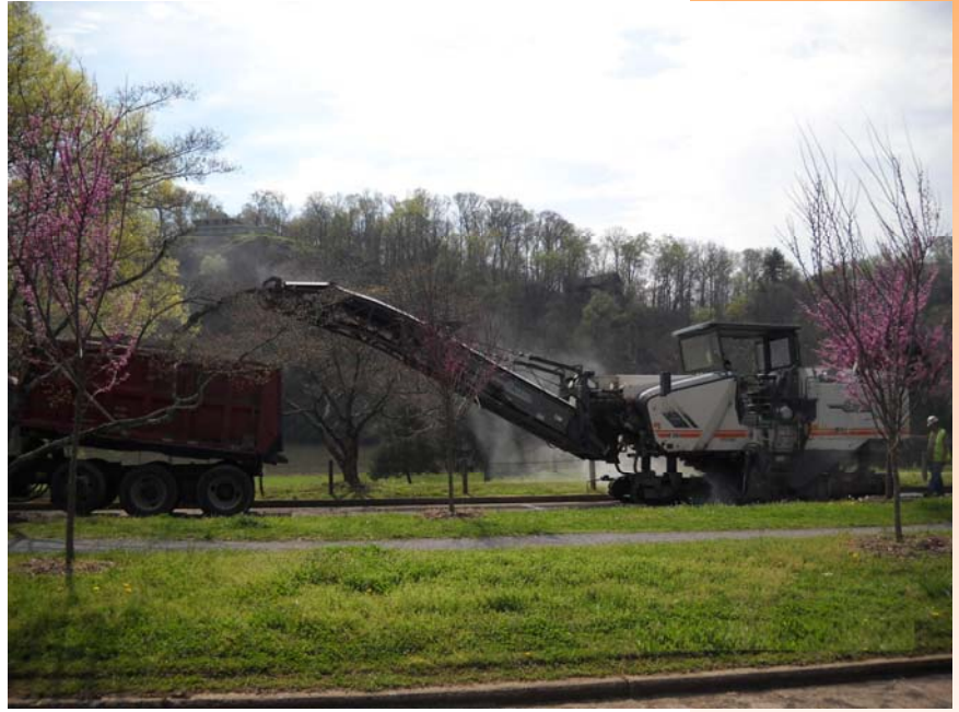
Milling Along Cherokee Boulevard
