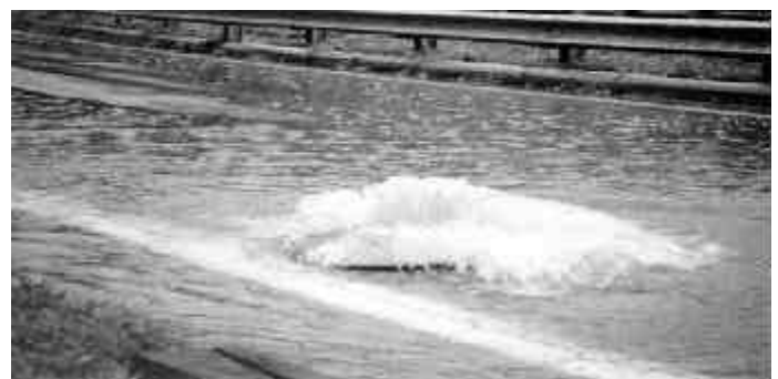
When sanitary sewer systems are not maintained, or lack adequate capacity, discharges of raw sewage and industrial wastewater can occur and potentially endanger the public and environment. (U.S. EPA photographs.)
