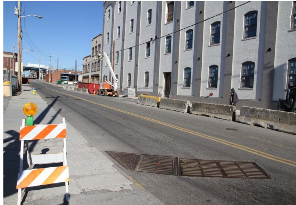
Central Ave at RR looking north toward Depot St
