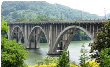
Henley Street Bridge, Knoxville TN
