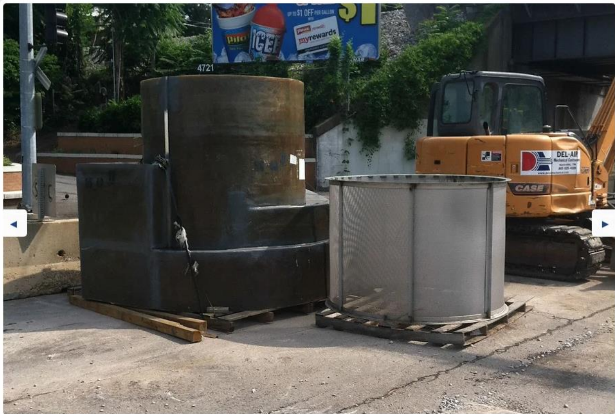
June 19, 2015: Progress Strainer Basket for New Water Quality Unit
