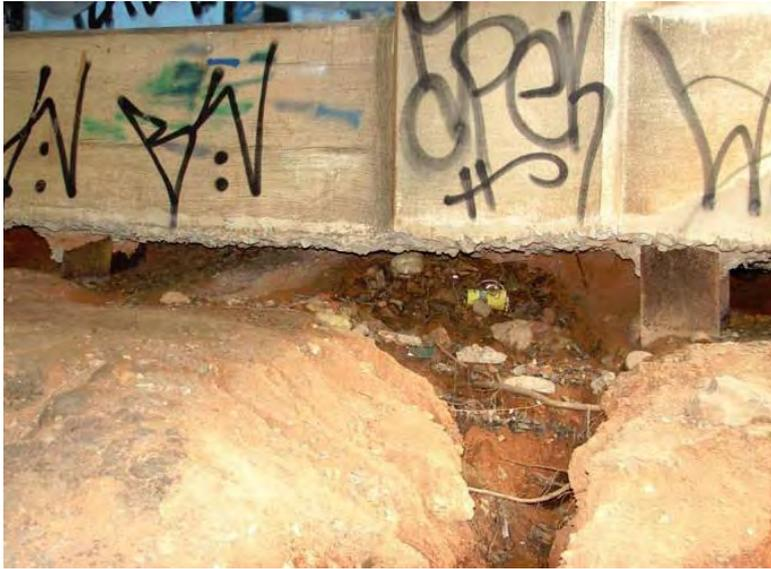
Exposed Pilings Beneath the Ed Shouse Drive Bridge
