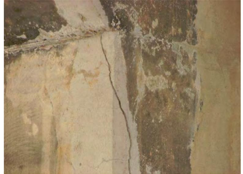
Vertical Cracking Along an Abutment of the Sutherland Avenue Bridge
